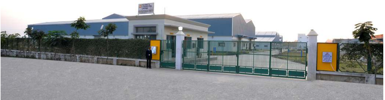
EHV Plant at Sitarganj
